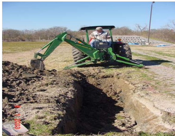
Figure 3.12 Construction of trenches at ALF site
