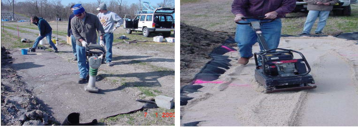
Figure 3.14 Compaction of trenches at ALF site
