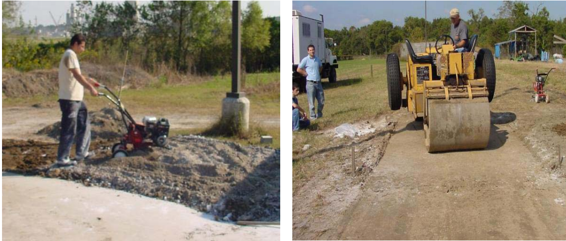
Figure 3.9 Construction of ALF sections
