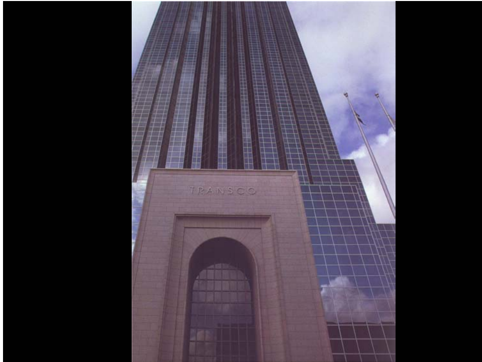
Figure 6. The Entrance to the Tower
