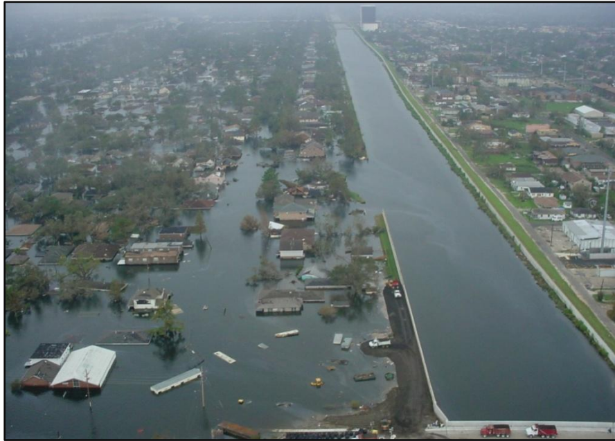
Figure 7 – 17 th Street Canal levee breach. The flooded Lakeview neighborhood is on the left of the canal. Courtesy of the U.S. Army Corps of Engineers (Source: http://www.mvd.usace.army.mil/hurricane/KatrinaImages/Misc/DSC00033.JPG ).
