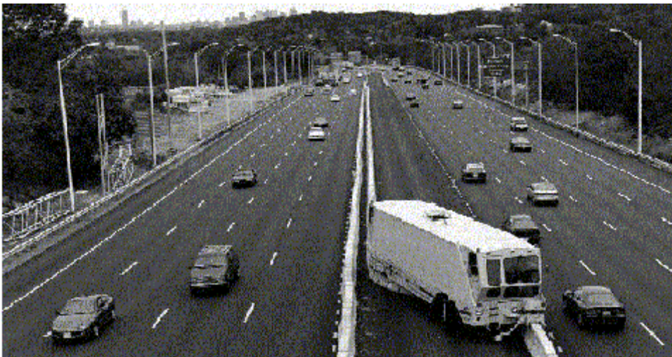
Figure 2-1 SE Expressway on I-93. (Photo by Massachusetts Highway Department)
