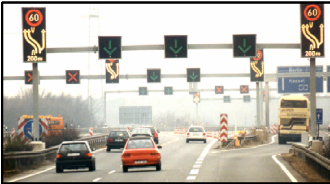
Figure 2-2 A tidal flow operation on the urban freeway including interchanges and it switched twice a day (VISUM-online, 2000).
