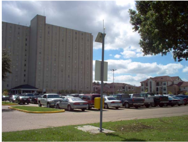
Figure 7. Kirby Smith parking lot
