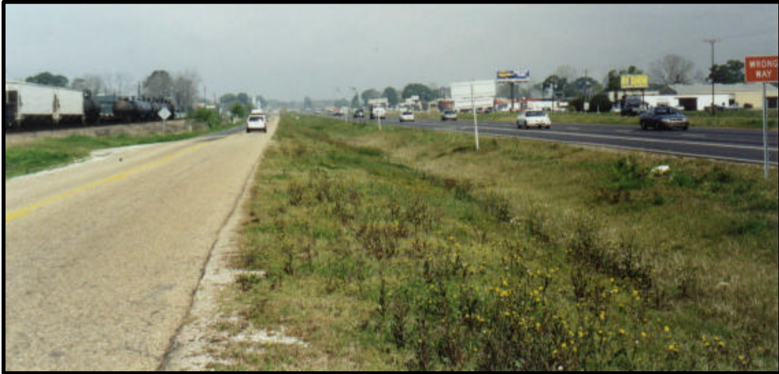
Figure 4.2 – Photo of US-90 with service road (By author)
