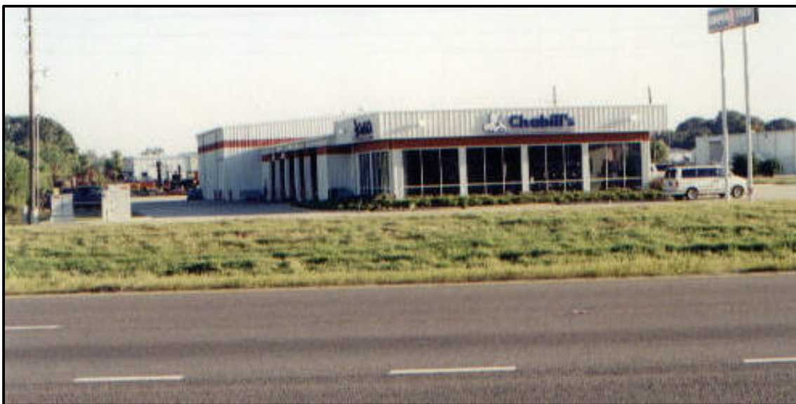
Figure 4.6 – Case study site 2 (Chabill's) photo. North and west elevation (By author)
