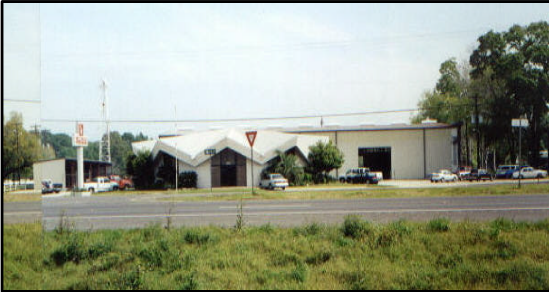
Figure 4.8 – Site case study site 3 (Tong Specialty). West elevation (By author)
