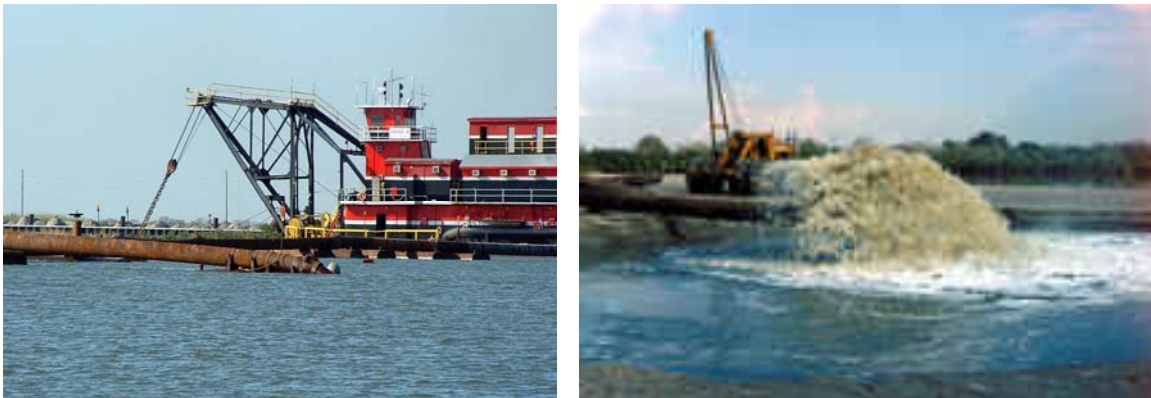
Figure 2-1 During hydraulic dredging to maintain navigation channels (left), a slurry of water and sediments can be pumped considerable distances and discharged at sites where sediments accumulate to form gently sloping marsh land (right).
